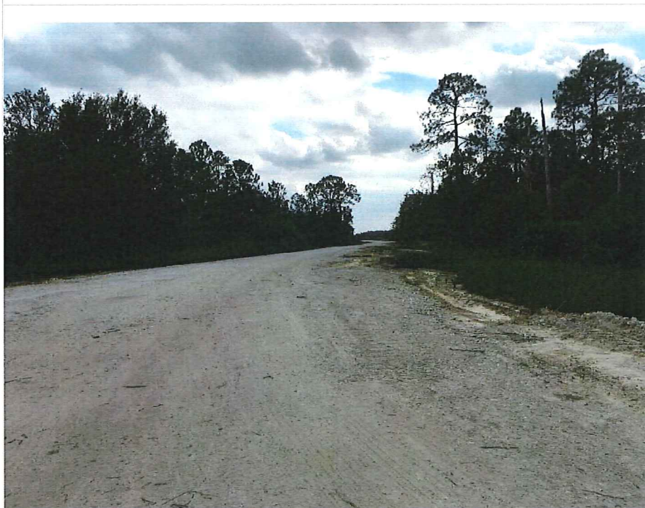
S'LY VIEW ALONG ACCESS ROAD FROM ARBORWOOD
