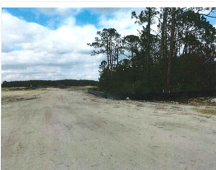
N'LY VIEW ALONG PARCEL 1
